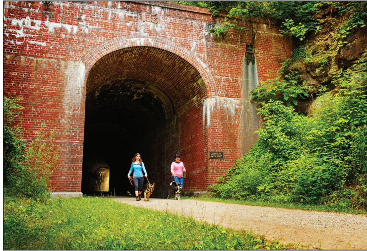
The former Baltimore & Ohio Railroad Tunnel No. 13 near Cornwallis is part of the 72-mile North Bend Rail Trail near Cornwallis. Hikers are welcome to take their pets as they travel across the 36 bridges and through the 10 tunnels that are part of the trail.
